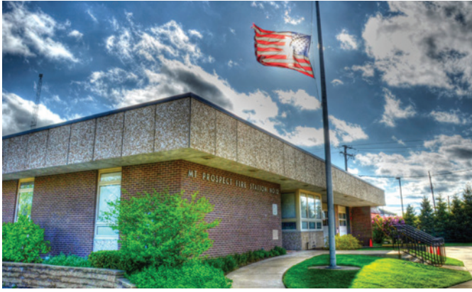
FIRE STATION 12 1601 W. Golf Road
