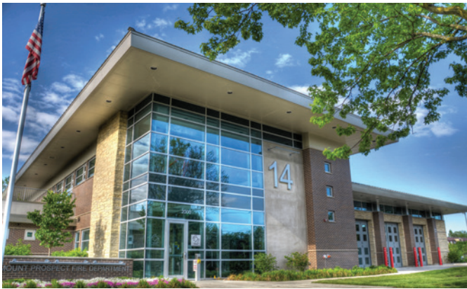
FIRE STATION 14 2000 E. Kensington Road
