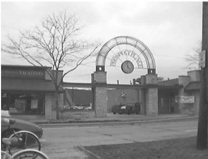
The pattern of land uses on the south side of the railroad tracks is cohesive, in terms of both physical structures and land uses.
