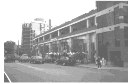
The idea of a multiple story parking deck in the downtown presents both opportunities and challenges.
