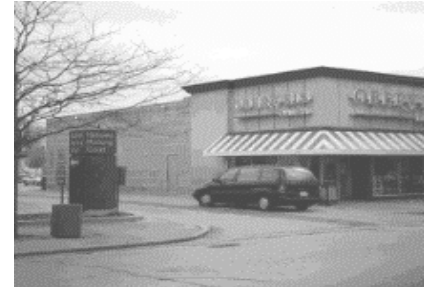
Parking lots should be at the rear or side of retail or entertainment buildings.
