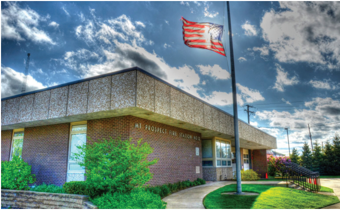
FIRE STATION 12 1601 W. Golf Road
