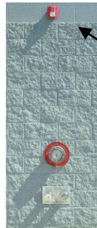
Outdoor strobe to be placed above fire department connection
