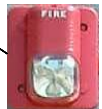
Outdoor strobe to be placed above fire department connection
