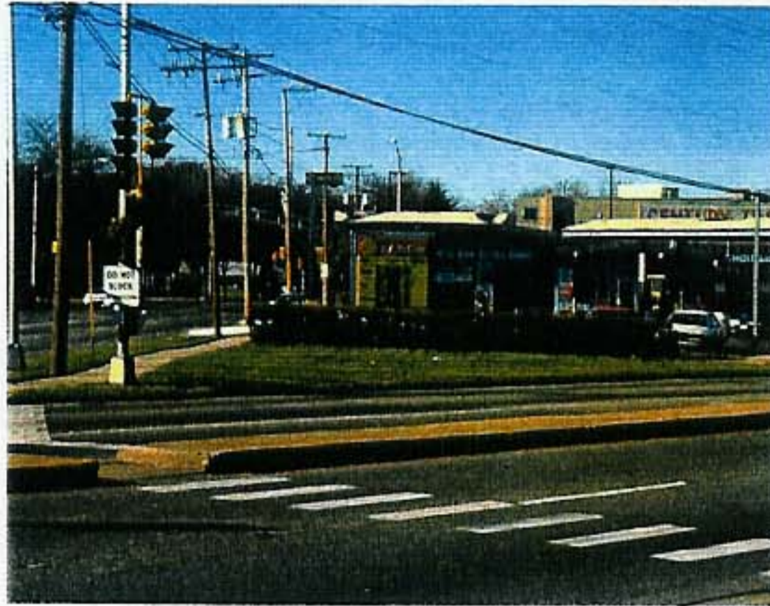
Looking west toward site nine (existing)
