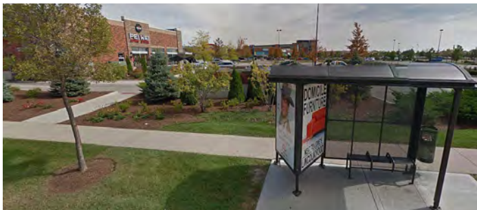
Construction of new sidewalks in gap locations, particularly to improve access to existing transit routes, is an eligible activity for ITEP funding.
