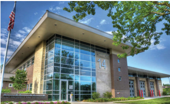
FIRE STATION 14 2000 E. Kensington Road
