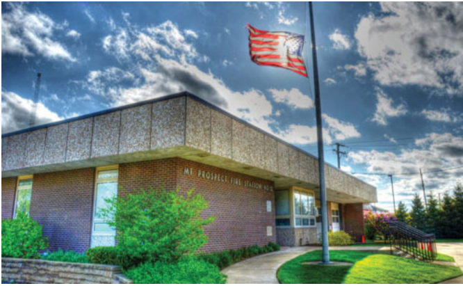
FIRE STATION 12 1601 W. Golf Road
