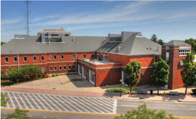
FIRE STATION 13 (Headquarters) 112 E. Northwest Highway
