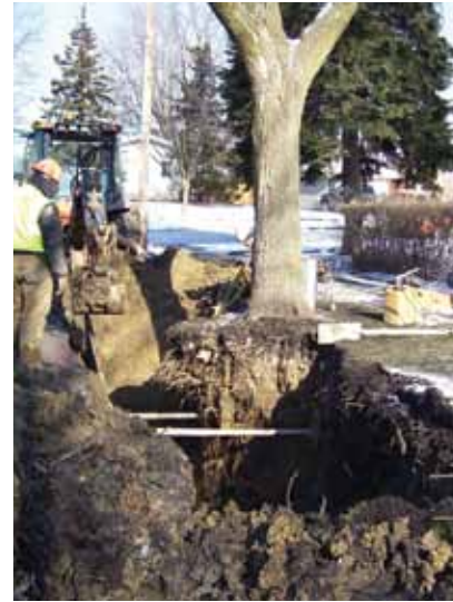
Photographs 3P-1a and 3P-1b. Left: Tree protection fencing installed to protect trees during construction activities on a Village street. Right: A parkway tree with roots severed during construction activities on Wilshire Drive in 2007.
