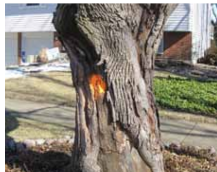
Photograph 3G-2. Defective Norway maple that was identified as part of the tree risk management program. The maple was scheduled for removal due to trunk decay and other defects.
