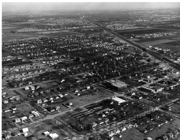
Photograph 3-2. Aerial photograph of the Village from 1956 showing the maturing elm population along streets. Dutch elm disease was just beginning to affect trees in the Chicago area at that time (Photograph courtesy of the Mount Prospect Historical Society).
