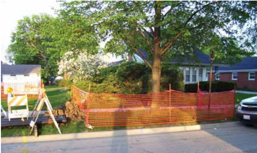
Photograph 3P-2. The Village Arboricultural Standards Manual and the Village ordinance provide specifications for the protection of trees such as the installation of tree protection fencing during construction activities.
