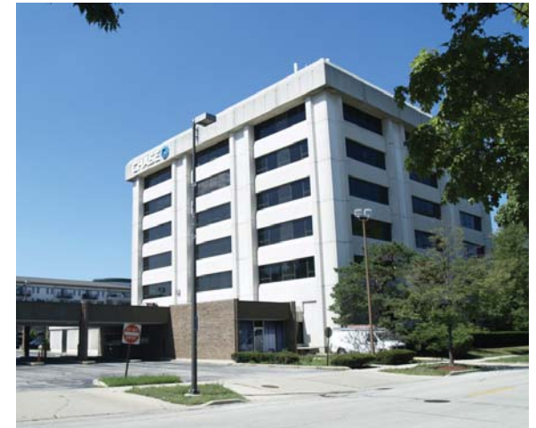
The six story Chase Bank building is across the street from one story single family homes.
