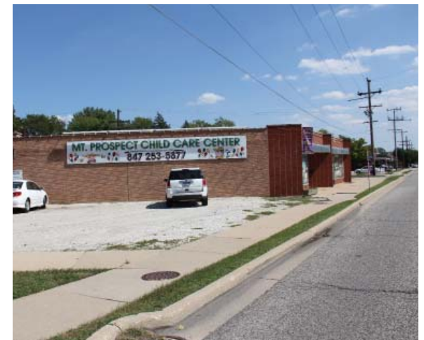
Streetscape in "fair" condition
