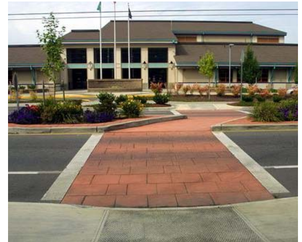
Landscaped median with pedestrian refuge
