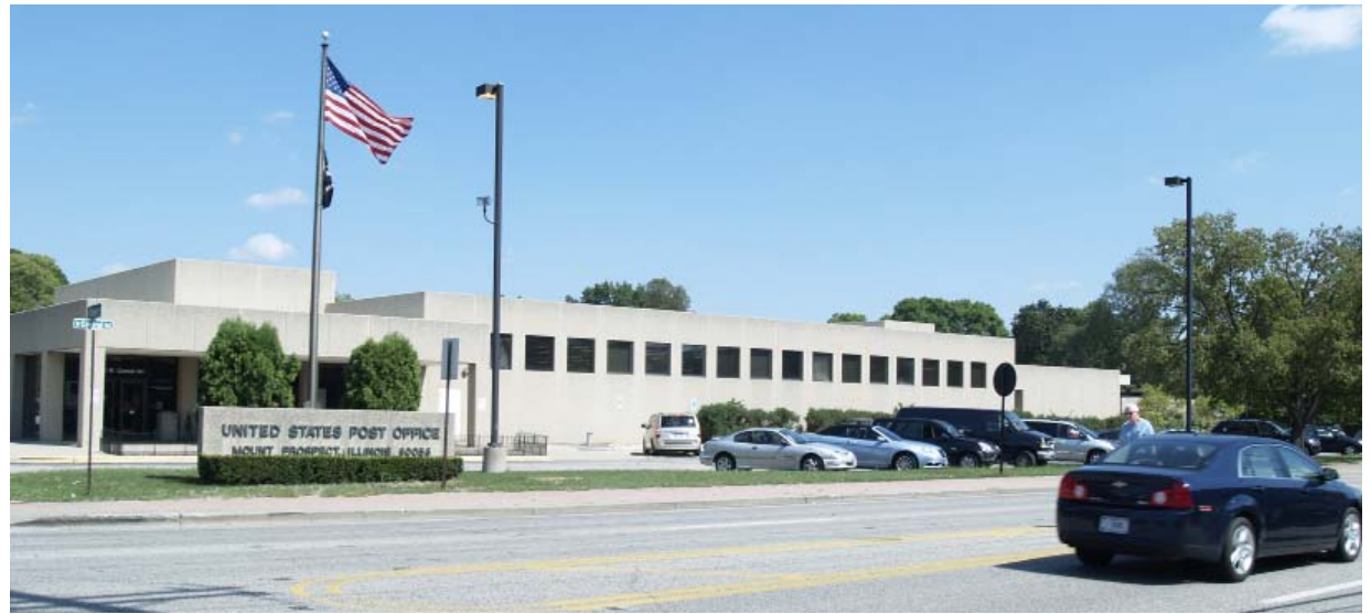
Existing Post Office Site
