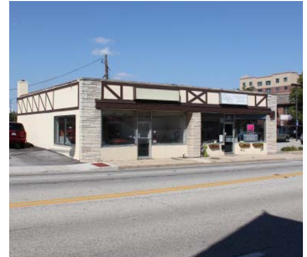
A few single story structures occupy the site today.
