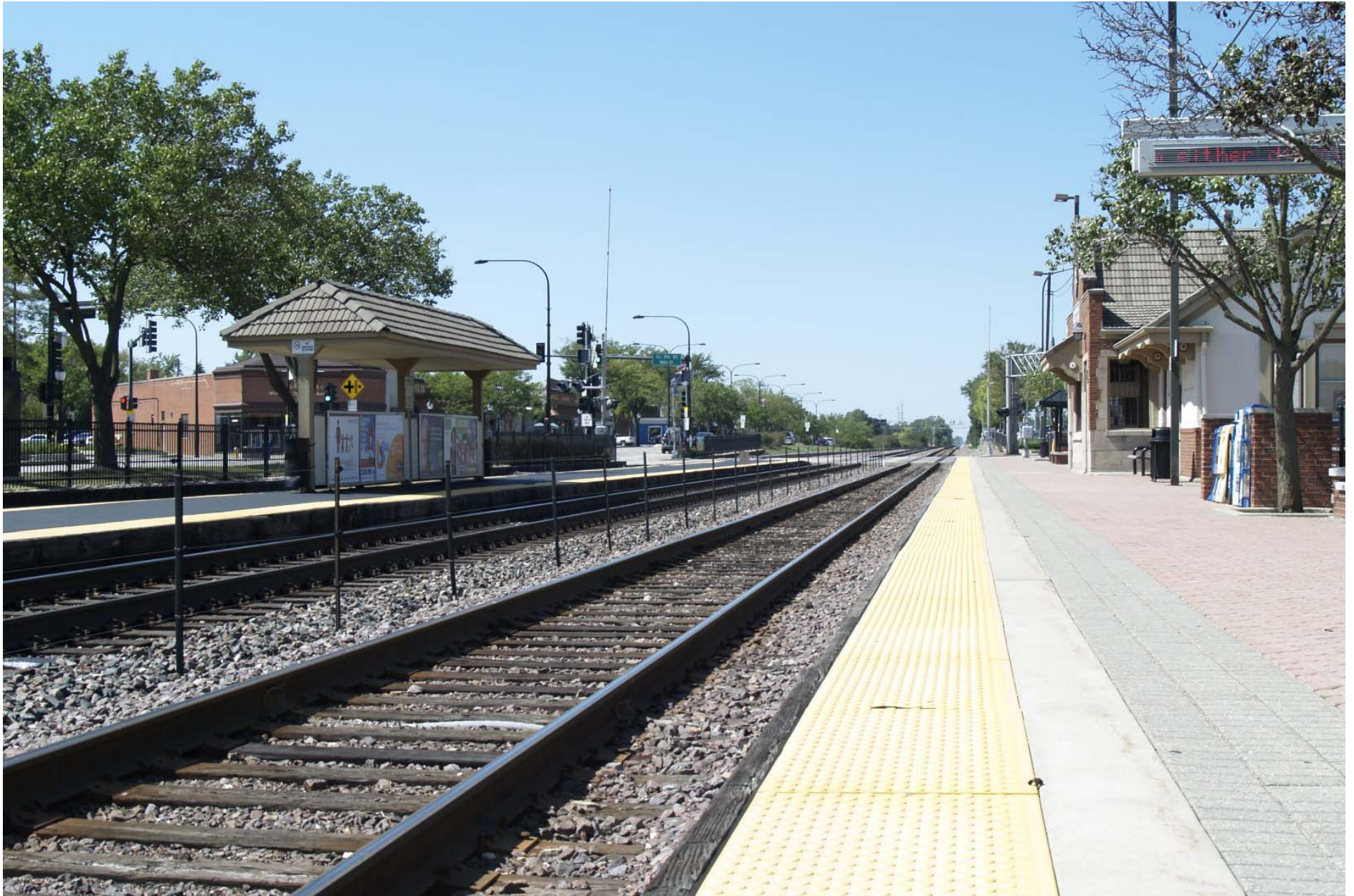
Mount Prospect Station along Metra's Union Pacific Northwest commuter rail line
