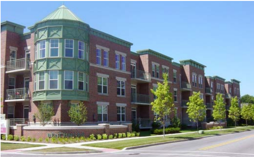
Multi-story buildings provide a transition from the Downtown core
