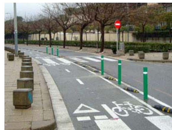
On-street bike lane with flexible plastic bollards
