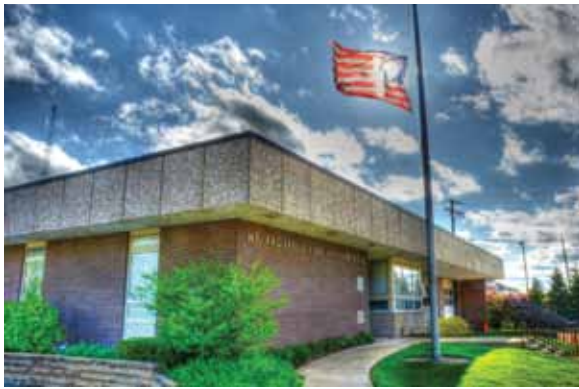
FIRE STATION 12 1601 W. Golf Road
