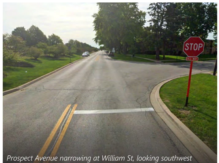
Looking northwest on Prospect Avenue at Emerson St
