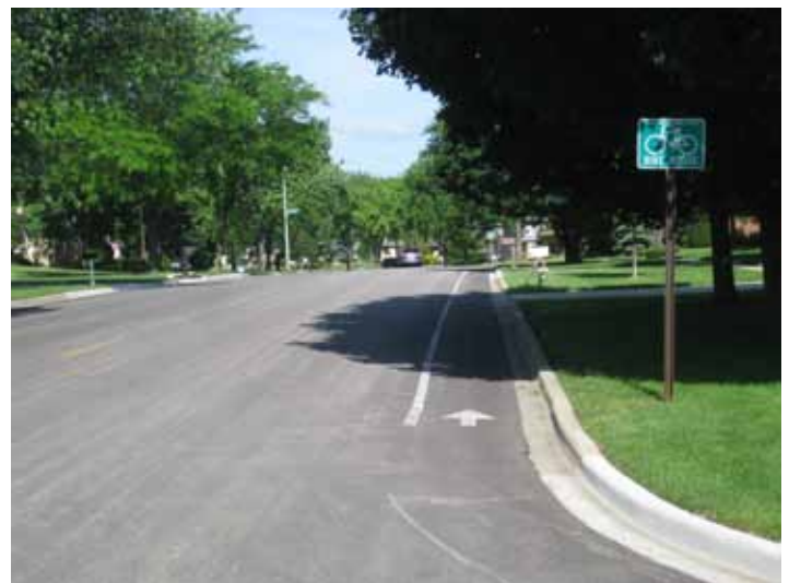
Figure 25: Weathersfield Way in Schaumburg provides one lane of travel and a bike lane in each direction. No parking is provided on street.
