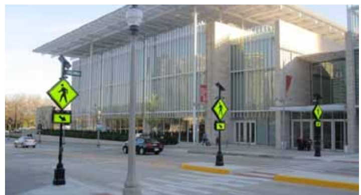
Figure 34: Example of an uncontrolled crossing
