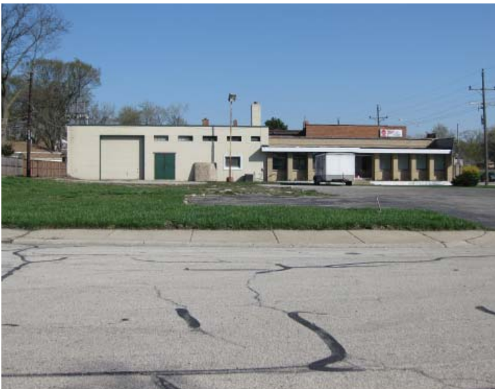
Northeast Corner of William St. and Northwest Hwy.
