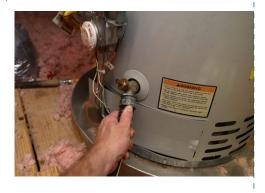
This process will likely cause several gallons of water to drain so have a bucket handy before you begin. A licensed plumber is recommended to properly drain piping, toilets, and traps to prevent freezing.
