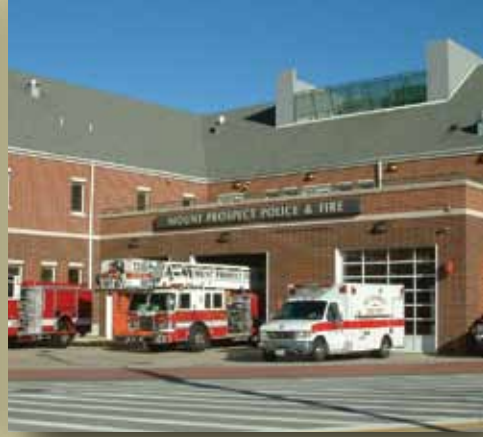
Fire Station 13 (HQ) 112 E. Northwest Highway
