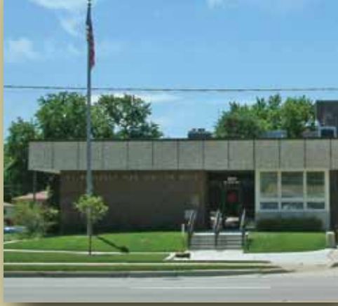
Fire Station 12 1601 W. Golf Road
