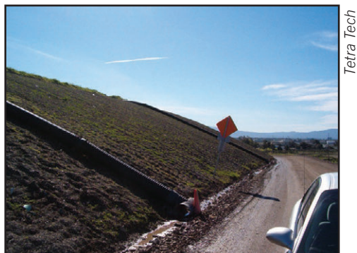
Figure 9. Slope drains to protect a hillside from erosion.
