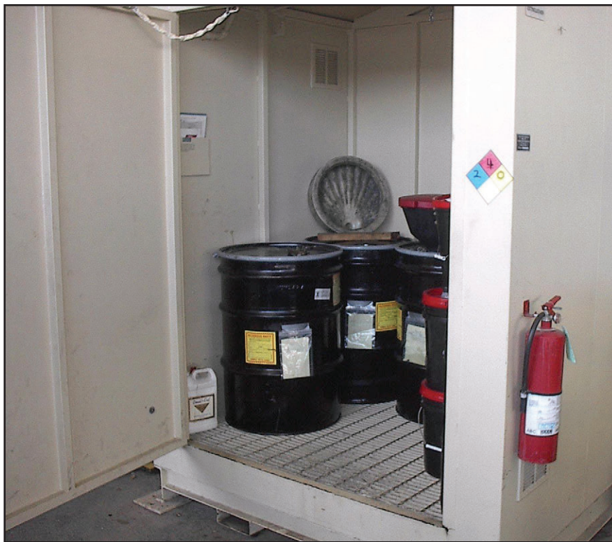
Figure 5. Minimize exposure by providing cover for potential contaminants.
