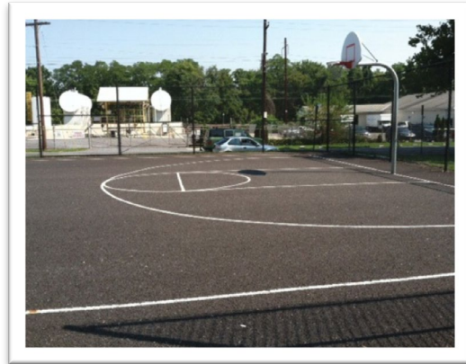
Porous pavement basketball court, Lancaster, PA Photo credit: Danielle Gallet, CNT
