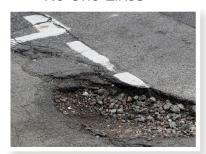
Pot holes in our roadways are caused by the expansion and contraction of water after it has entered into the ground under the pavement. When water freezes, it expands. Pot holes occur when snow and ice melt as part of seasonal freeze-thaw cycles, The reoccurring cycle of snow and ice melting throughout the winter season is the primary reason why potholes rear their ugly head on our streets.
