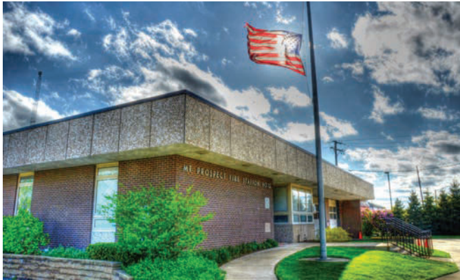
FIRE STATION 12 1601 W. Golf Road
